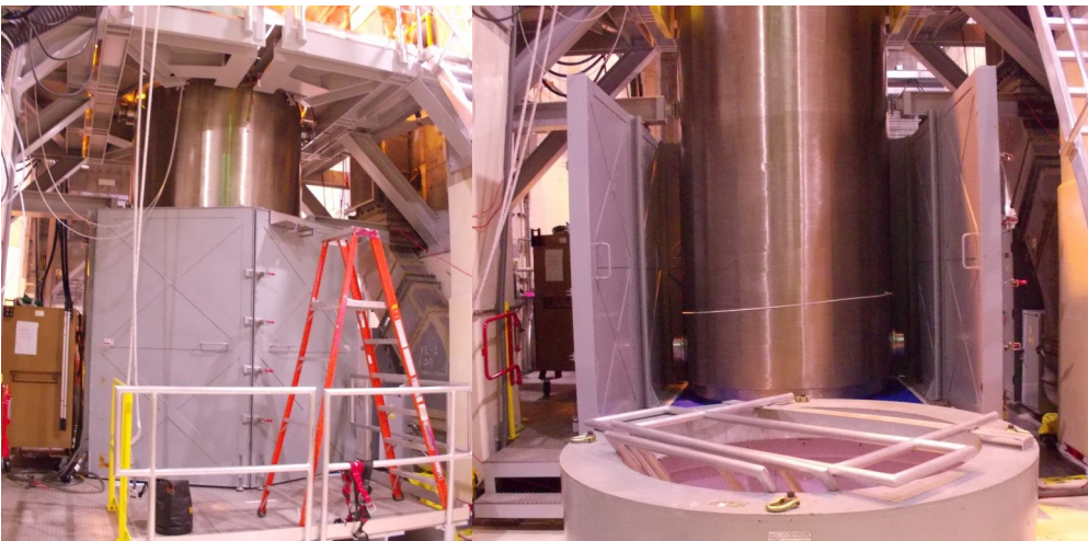
Millstone - Lower transfer cask shielding. Primarily provides neutron reduction and has large doors for bringing in and taking out transfer cask.
